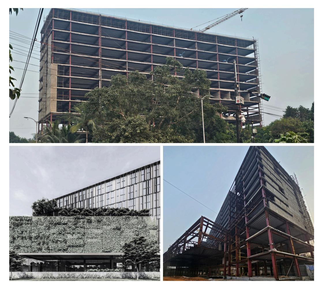
A complex structure with large cantilever, roof top pools, triple height ball rooms and a an added floor.
